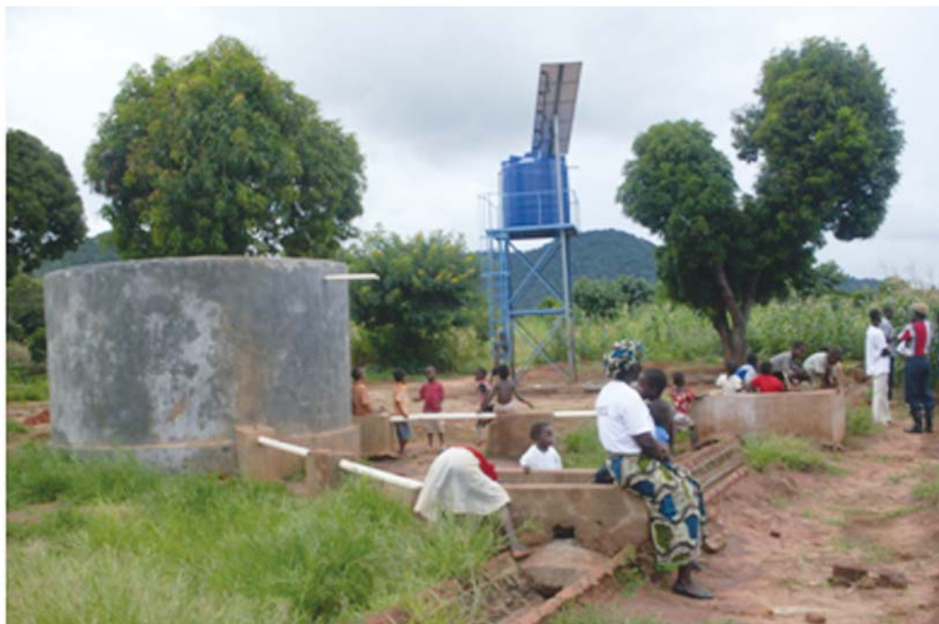
Photovoltaic panel, tank and storage facility for Mzee DRR Club
