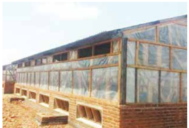
Plate 14 The initial pilot solar fish dryer was smaller (left) that was later enlarged and modified (right) following lessons learnt and increased demand from women fish processors from Kachulu beach, Lake Chilwa in Zomba. Photo credit: Welton Phalira and Precious Mwanza.
