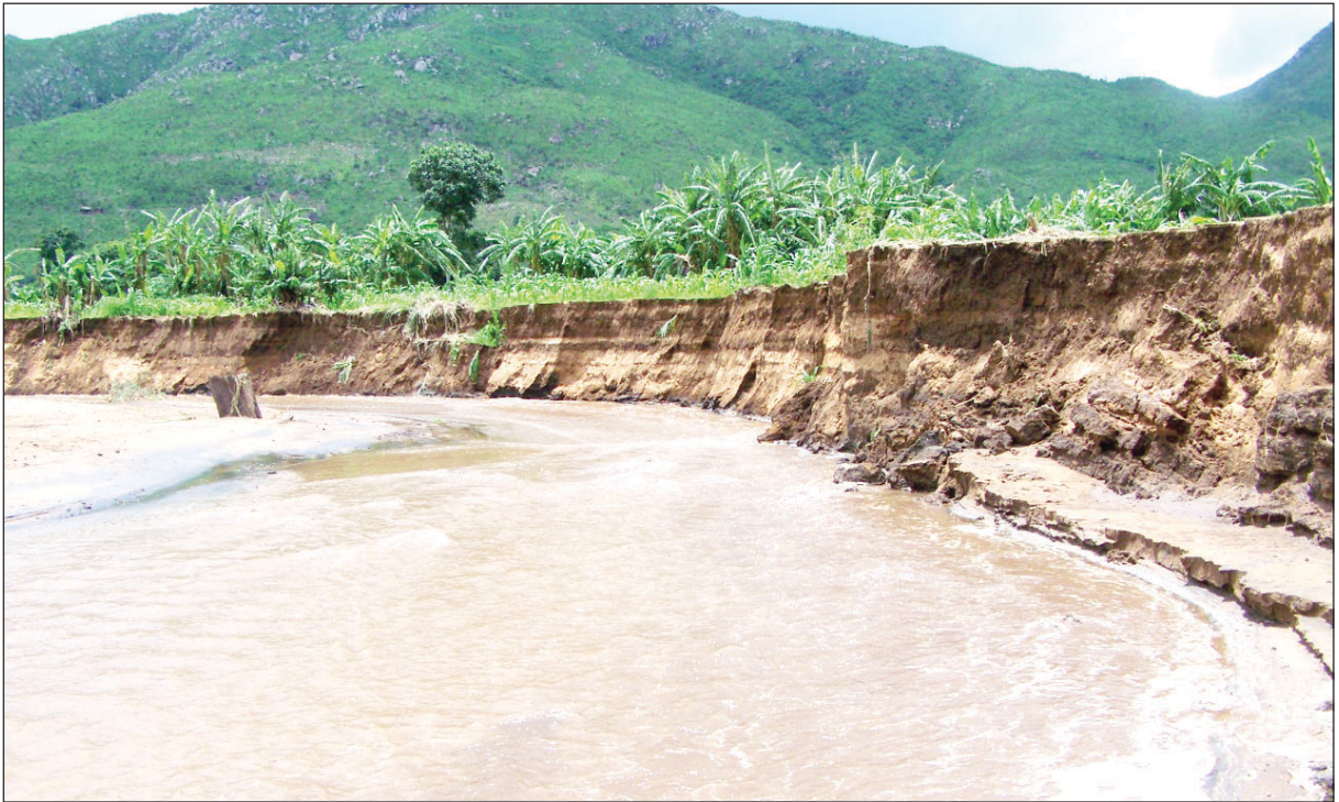
Environmental degradation caused by flooding
