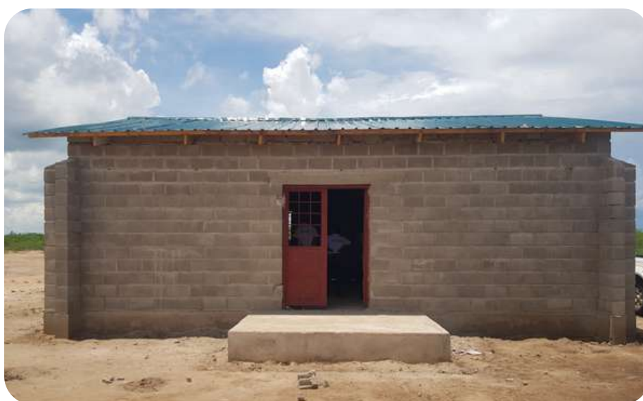
Front view of the Salt Storage Unit, 2023
